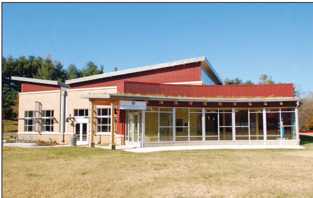
A green community center: The new Dr. Wesley Grant Sr. Southside Center uses a geothermal HVAC system, skylights and a living roof (floor plan below).
