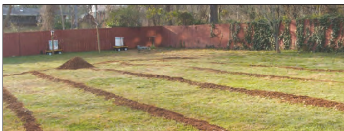
Figure 4: Piping laid out like a “vertical Slinky” is placed in trenches for this geothermal loopfield.
