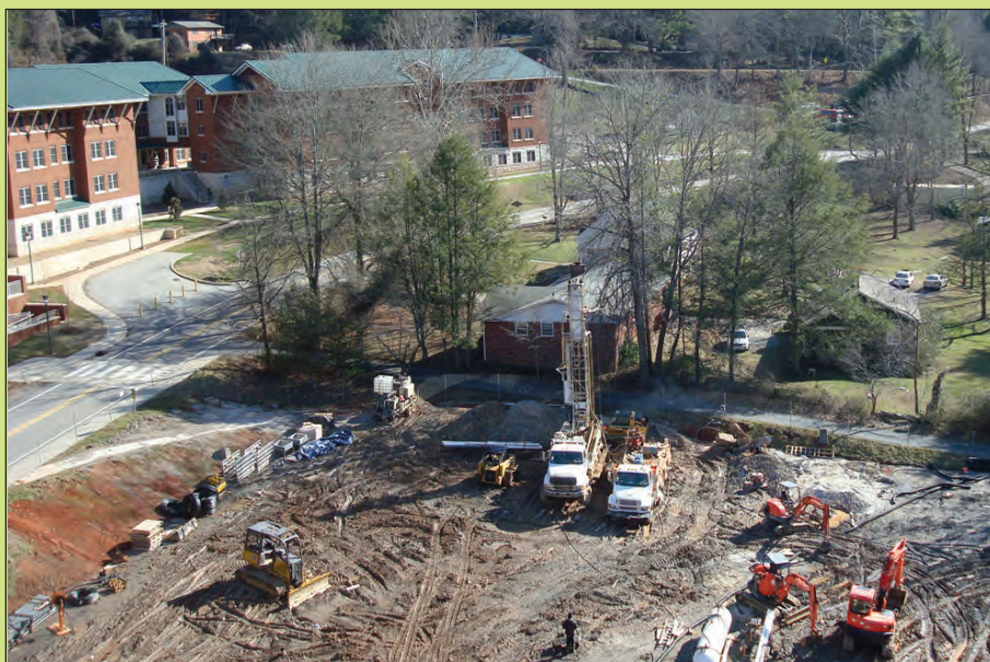
Earth warmed: While Warren Wilson College has earned national recognition for its green initiatives, other regional institutions have set to work too, such as this geothermal-well system under way at Western Carolina University.
