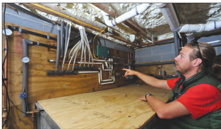
Systematic: A solar-thermal installation supplies the radiant-heat floor system, above, one of several features that help achieve net-zero energy use, says homeowner Ryan Lubbers.
