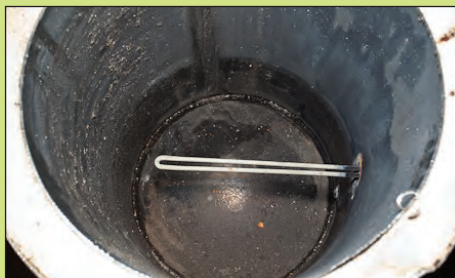
Electric Storage Water Heater After 90 Days Using Softened Water
