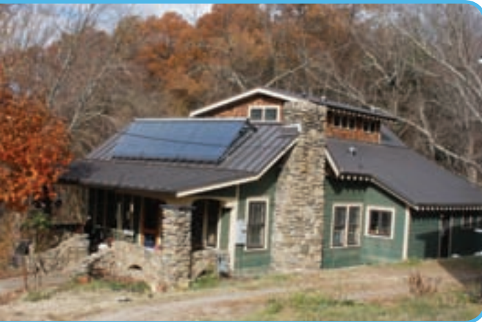
Gaining control: Water heated in an evacuated tube system on the roof provides radiant in-floor heat organized in four zones in the house, as Blake Esselstyn explains. Natural gas provides backup on cloudy days. Solar collectors, a second-floor addition, and original rock work are visible at this updated 1920s cottage.
