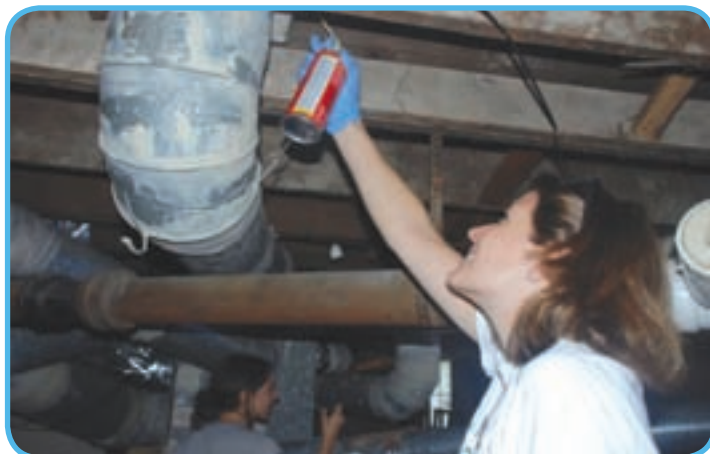
Energy saver: An AmeriCorps Member uses a can of spray foam to air seal large holes under the floor to save energy and improve comfort during "Project Energize."
