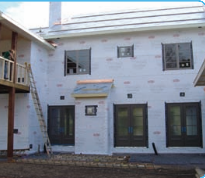
Wrapped up: Careful application of the housewrap helps ensure a tight home that will last for years.
