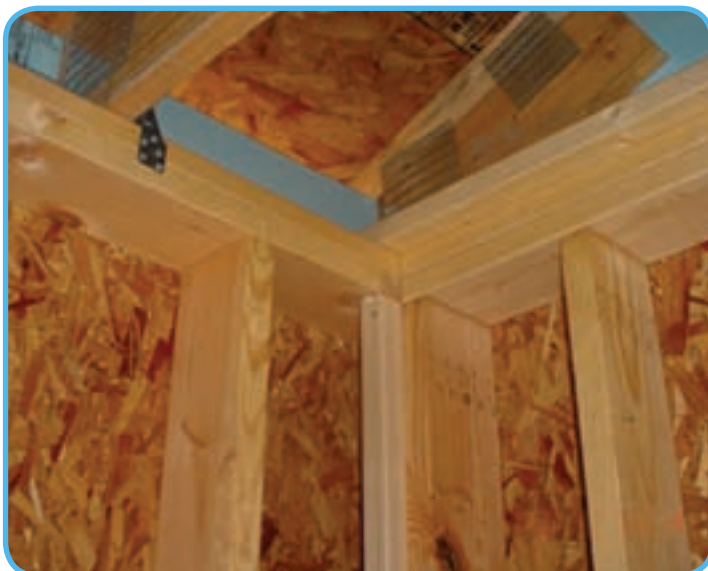
Details: Two-stud corners, raised-heel trusses and proper blocking are important construction details of ENERGY STAR home.
